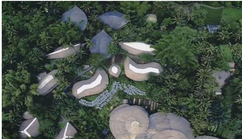
Figure 1. Green School in Bali
